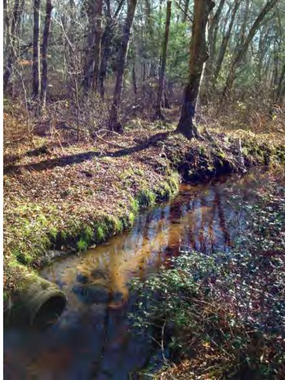
18" RCP discharge into Effluent Brook.
